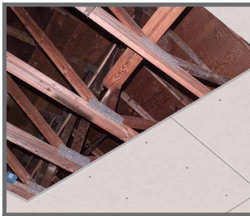
A Install Ceiling
