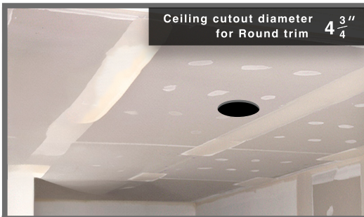
C Cutout opening for light install.
